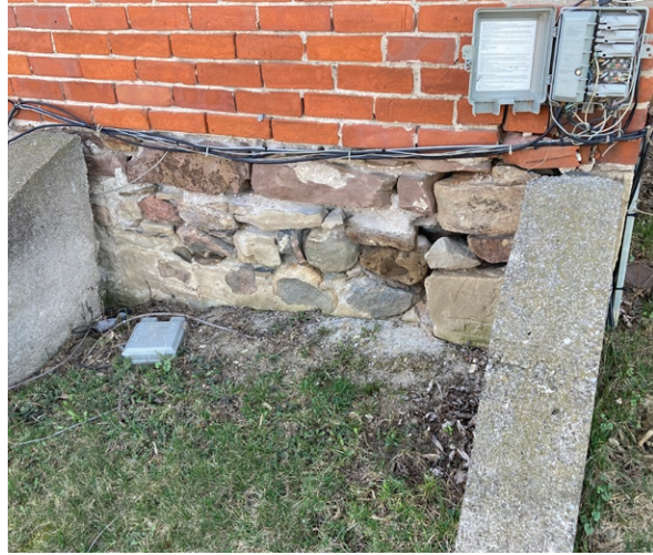
Severe deterioration of foundation pointing (ERA, 2023).
