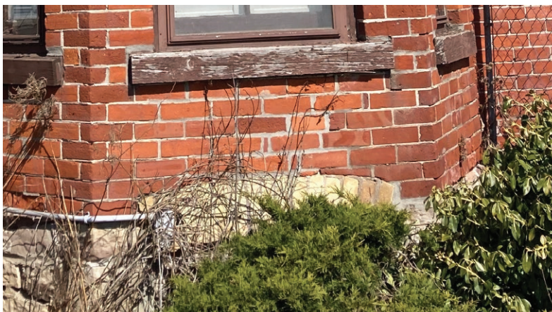
Evidence of step cracking below the bay window sill, infilled with unsympathetic mortar (ERA, 2023).
