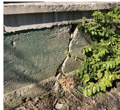
Cracking on the porch's stone foundation (ERA, 2023).
