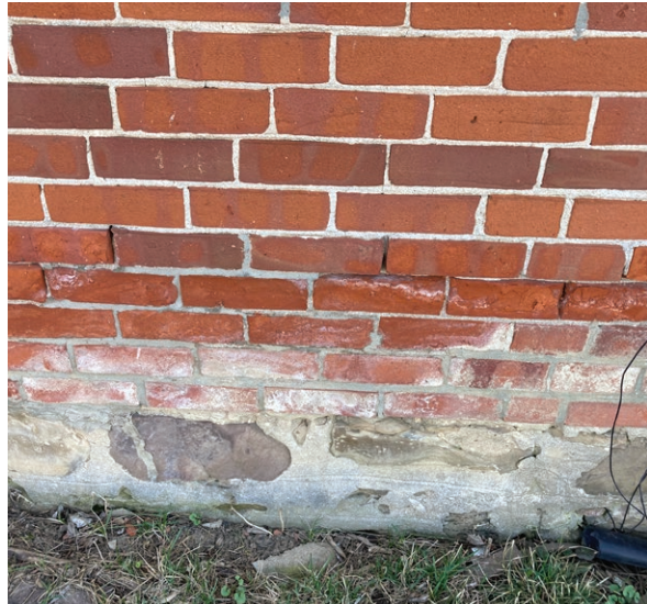
Efflorescence and spalling (ERA, 2023).
