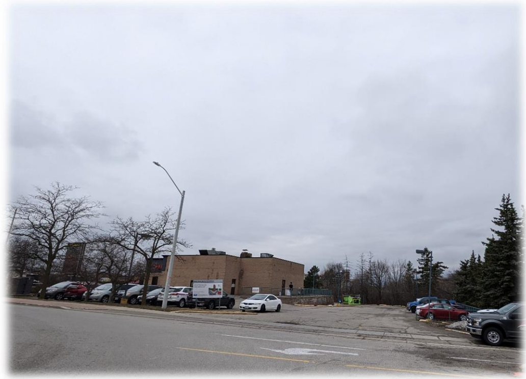
View from the Southeast
