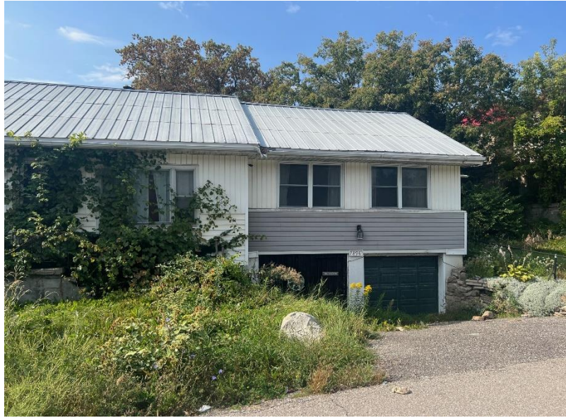
Street view looking West
