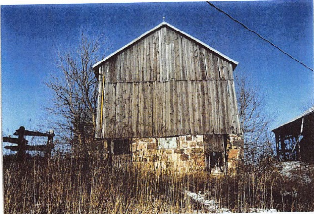
Figure 6 Robinson Barn as it stood in Caledon, Ontario 121
