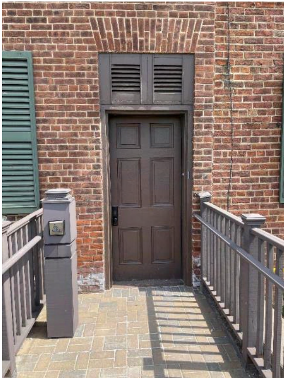
Figure 18: Main House - Existing Barrier Free Entrance
