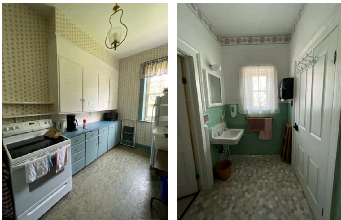
Figure 25: Existing modern kitchen on ground floor and washroom on second floor where lift could potentially be located
