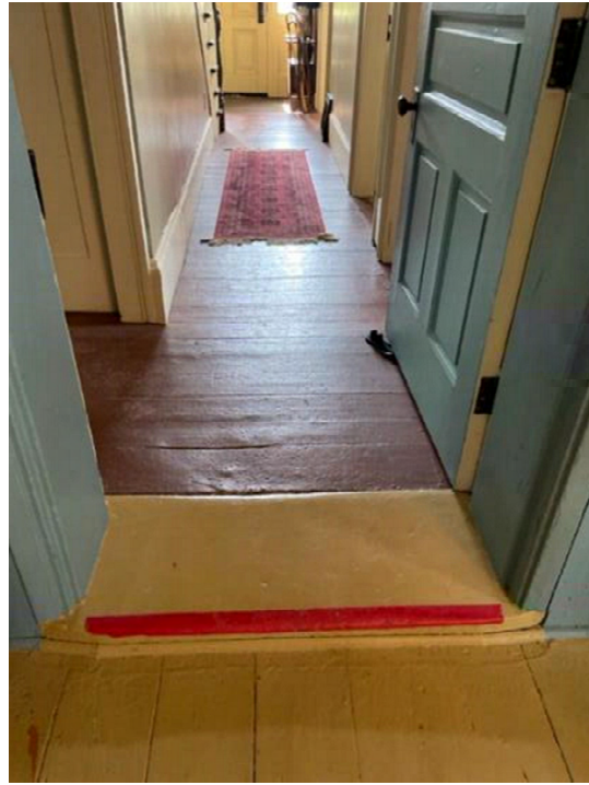
Figure 21: Main House - Step from Farm Kitchen
