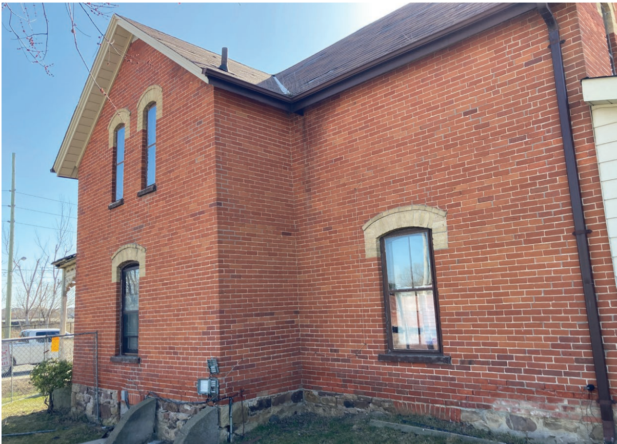
North elevation of the farmhouse
