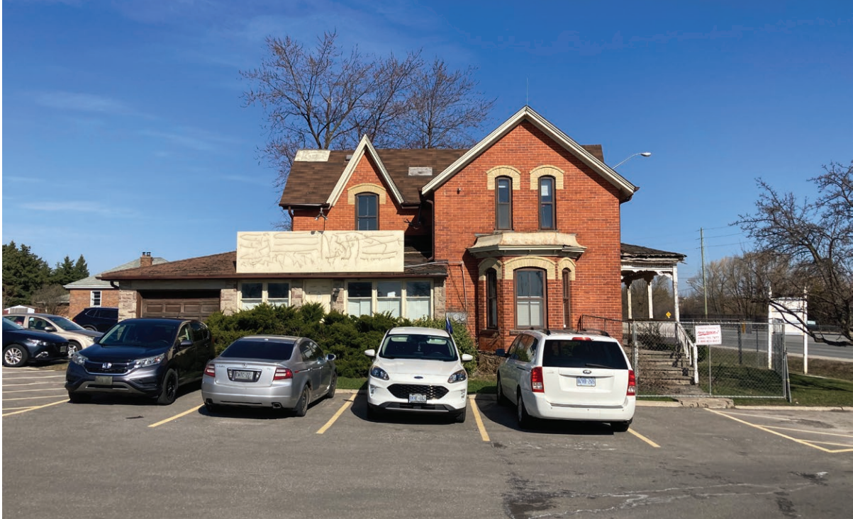
South elevation of the farmhouse (ERA, 2023).
