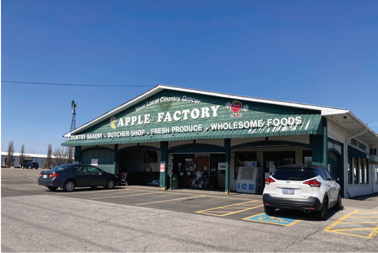
The Apple Factory building at 10024 Mississauga Road on the Site (ERA, 2023).
