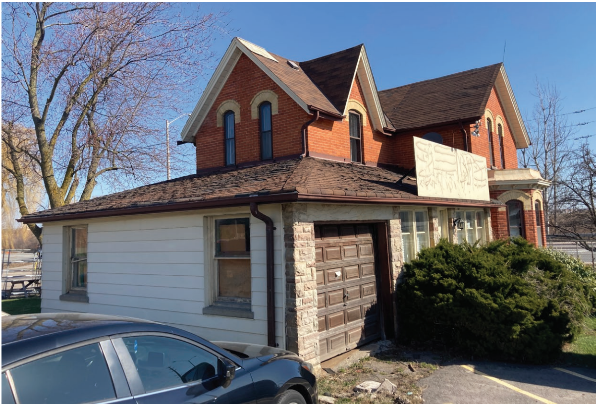
South and west elevation of the farmhouse (ERA, 2023).
