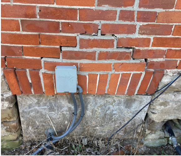
Step crack above basement window (ERA, 2023).
