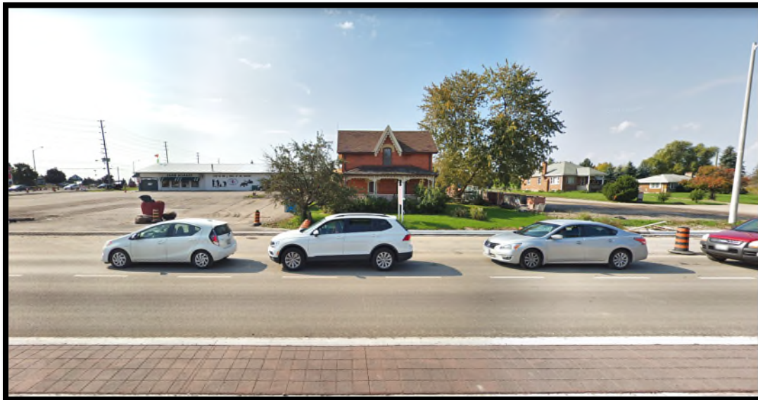
Figure 6: The brick residence in centre with The Apple Factory market building in the background on the left and the two residences located on the right side of the brick residence at 10042 (right) and 10054 (extreme right) on Mississauga Road. (Google Map, 2018)
