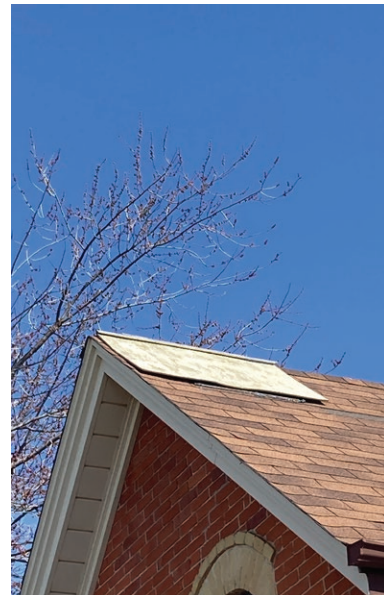
Former opening for chimney stack, with a temporary cover (ERA, 2023).
