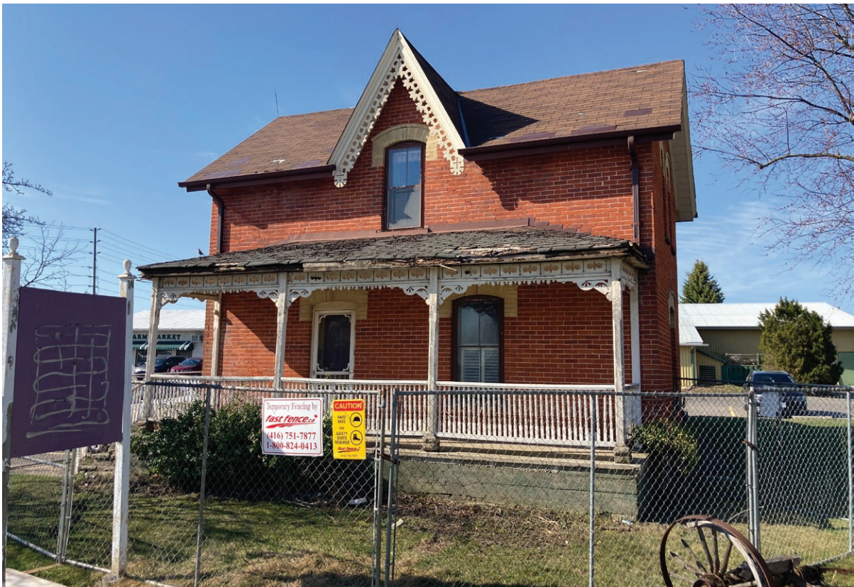
East elevation of the farmhouse (ERA, 2023).
